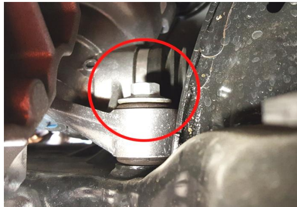
13. Driver side steering rack bolt.
